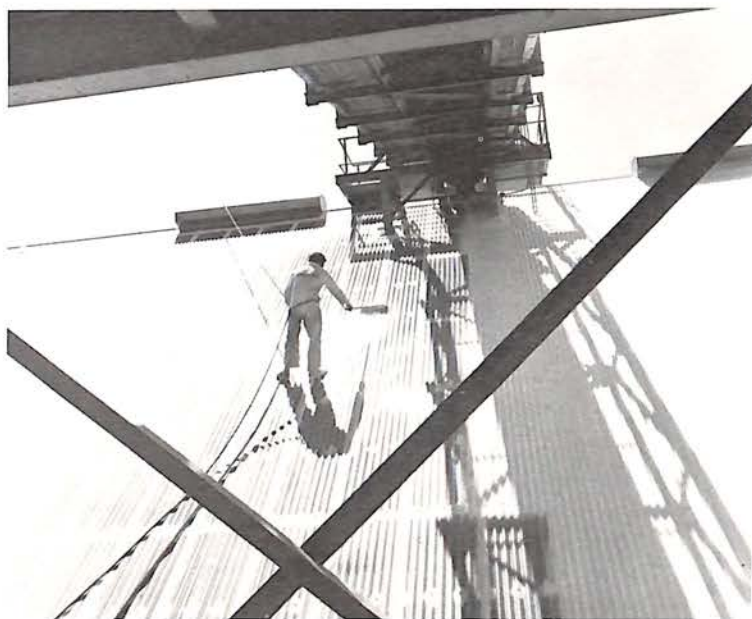
Sealing a silo before fumigation with carbon dioxide to destroy stored-grain pests.
