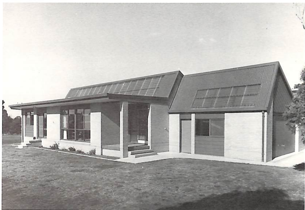
The CSIRO low-energy house in Melbourne, designed to reduce energy consumption. Its special features include solar energy systems for heating and cooling, good insulation, and wide eaves to protect against summer sun but allow entry of winter sun.
