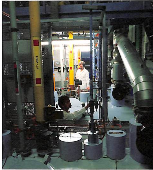
Engineering staff carrying out routine maintenance work on part of the liquid waste treatment plant at ANAHL. Heat is used to destroy any potentially harmful disease organisms that may be present in the waste.
