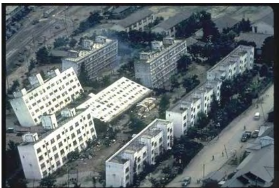
Buildings toppled by soil liquefaction in the 1964 earthquake at Niigata, Japan.
