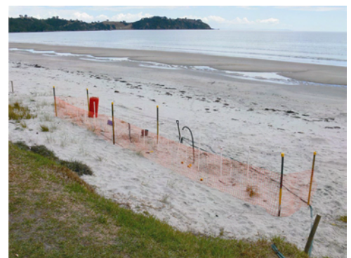
In 2008 Lithic Australia Pty Ltd constructed a 15m long backstop wall on Onetangi Beach, Waiheke Island, NZ, as a trial for Auckland City Council. The wall was built by injecting CIPS deep into the sand while the beach was being used by the public. When the work was finished the injection pipes were removed and the beach returned to its original condition.
