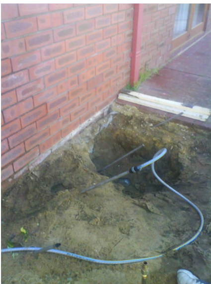
Injecting CIPS beneath the wall of a house in Perth, WA.
