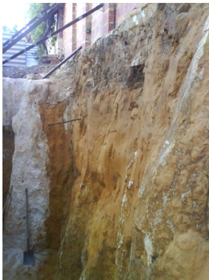
5m high face of an excavation at Fremantle, WA. The white material is limestone rock and the brown material is sand strengthened with CIPS by Earth Bond Solutions PL.
