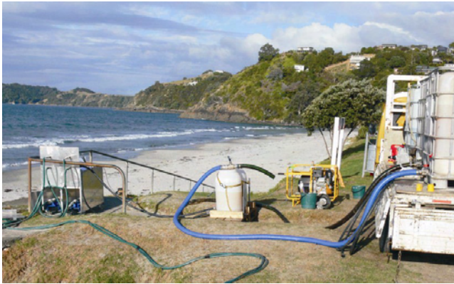
Injection pumps, hoses and CIPS solution tanks during construction of the below-surface backstop wall on Onetangi Beach, Waiheke Island, New Zealand.
