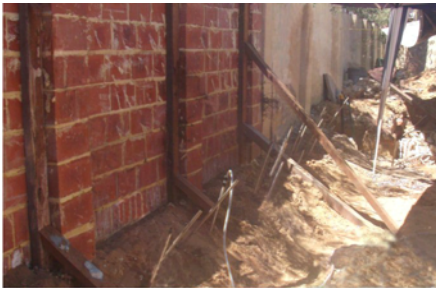
Injecting CIPS beneath the rear fence using multiple injection lances.
