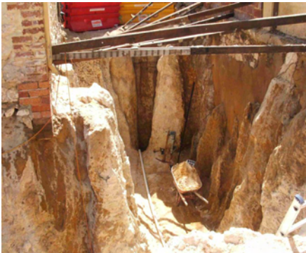
The completed excavation. Several white/cream coloured limestone pinnacles stand around the excavation. The CIPS-treated brown sand can be seen in the excavation face on the right.
