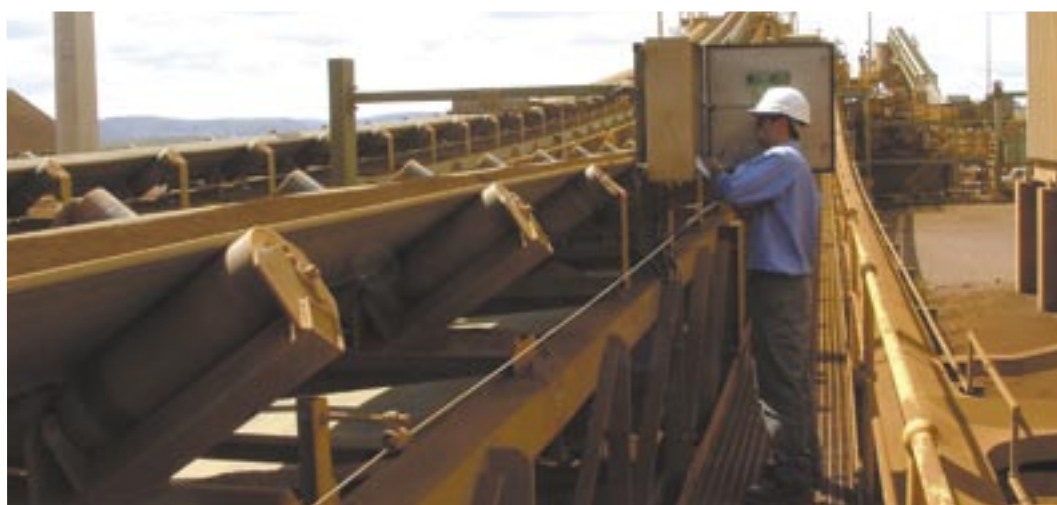
Tarek Kazzaz commissioning the low frequency microwave moisture analyser at an iron ore operation in Western Australia. Photo: Daniel Bennett
