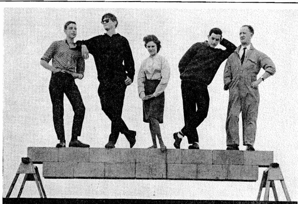
The Division of Building Research is investigating the use of epoxy resins as materials for binding together concrete blocks.
