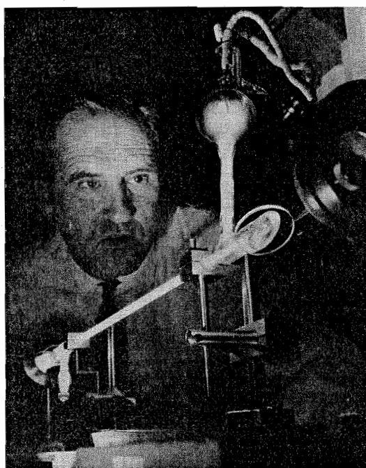
Above. Dr. J. V. Ramsay of the Division of Physics with a continuous-wave helium-neon laser.
